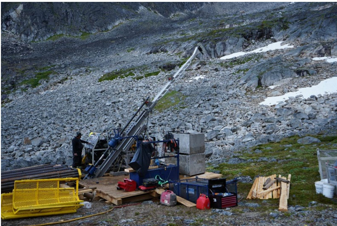
Figure 1. First hole being drilled at pad 1, Netazul Mt, Hazelton property, Smithers, BC
